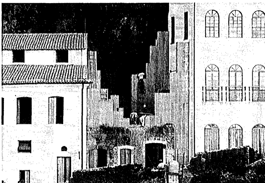
Restoration of Misericórdia Slope, Salvador, Bahia, 1987. Behind the remains of the old wall, buttresses reinforce the neighbouring houses and form the 'Bar of the 3 Arches'.
